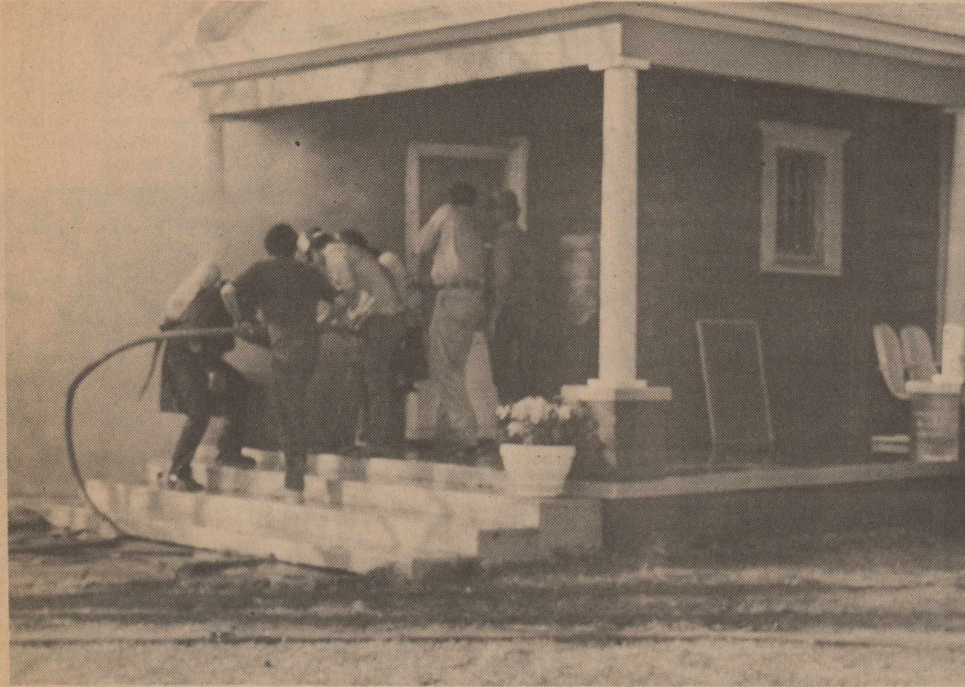
FIRE AT CUMMINGS HOME --The home of Mr. and Mrs. Billy Cummings was gutted last Thursday afternoon and members of the fire department are shown trying to quench the hungry blaze which destroyed most of the bottom floor of the landmark which stands at the corner of 3rd & Main in Stratford. No injuries were reported in the blaze although most of the furnishings in the home were destroyed.
