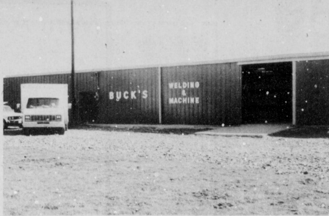
THE NEW 40x120 Buck's Machine and Welding Shop on FM 71 East will soon be ready for occupancy. Besides the
