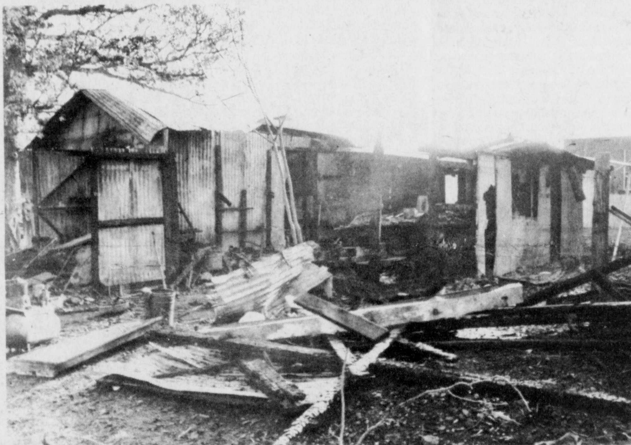
THE CHARRED remains of Russell Woodall's small engine repair shop are the result of a fire which totally destroyed the structure Thursday night, Janu-
