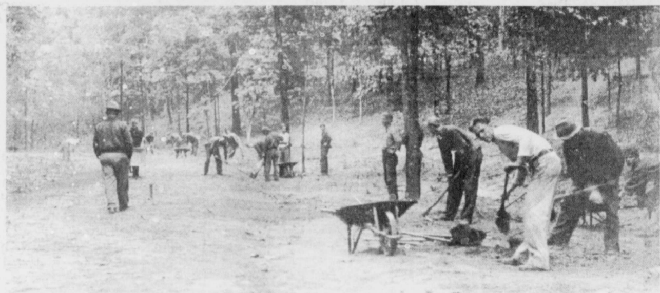
OLD PHOTO-this photograph of the CCC (Civilian Conservation Corps) show road work being done. The CCC was formed during the depression and provided work plus conservation efforts. This photo shows a roadbed being leveled with shovels and hoes.
