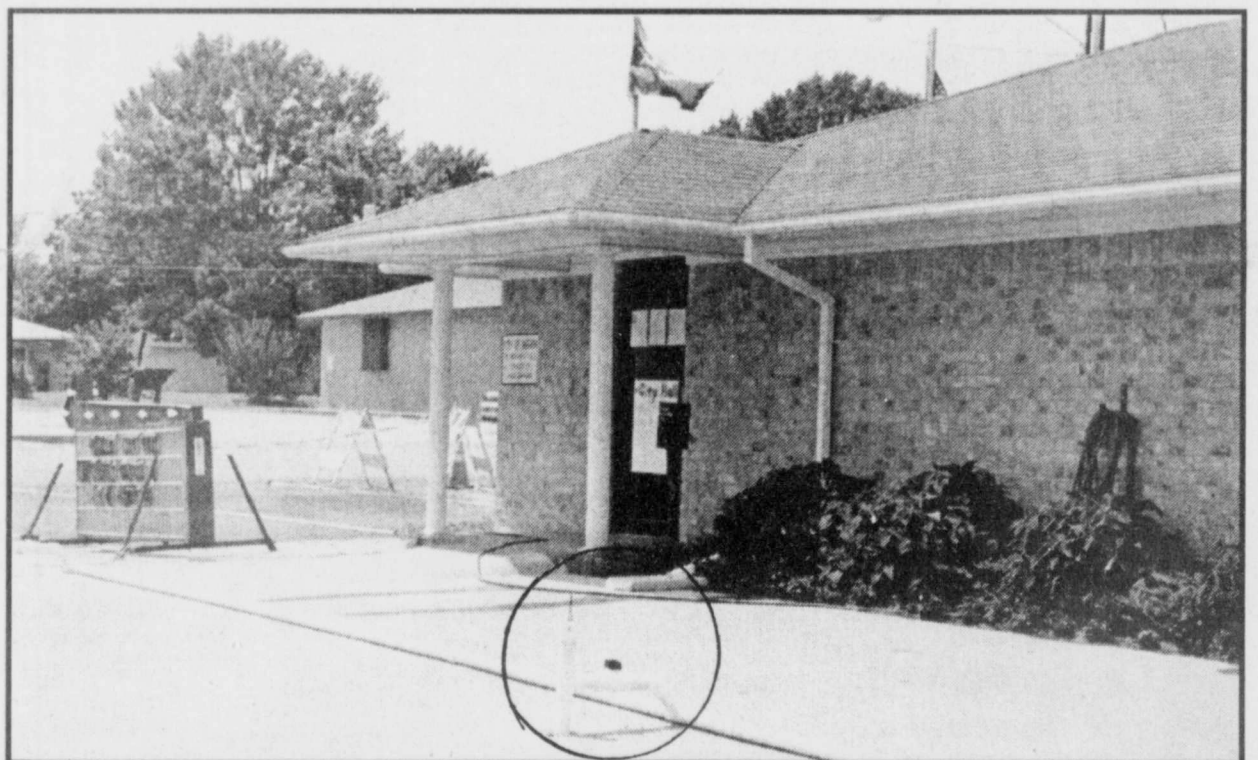
ALL CLEAR -The Texas Natural Resource Commission has given the green light for employees to move back to City Hall on Main Street next week. The circle on the above photo shows where traces of gasoline showed up after natural gas was gone. The TNRC has declared the level safe. (Staff Photo by Thomas Nichols)
