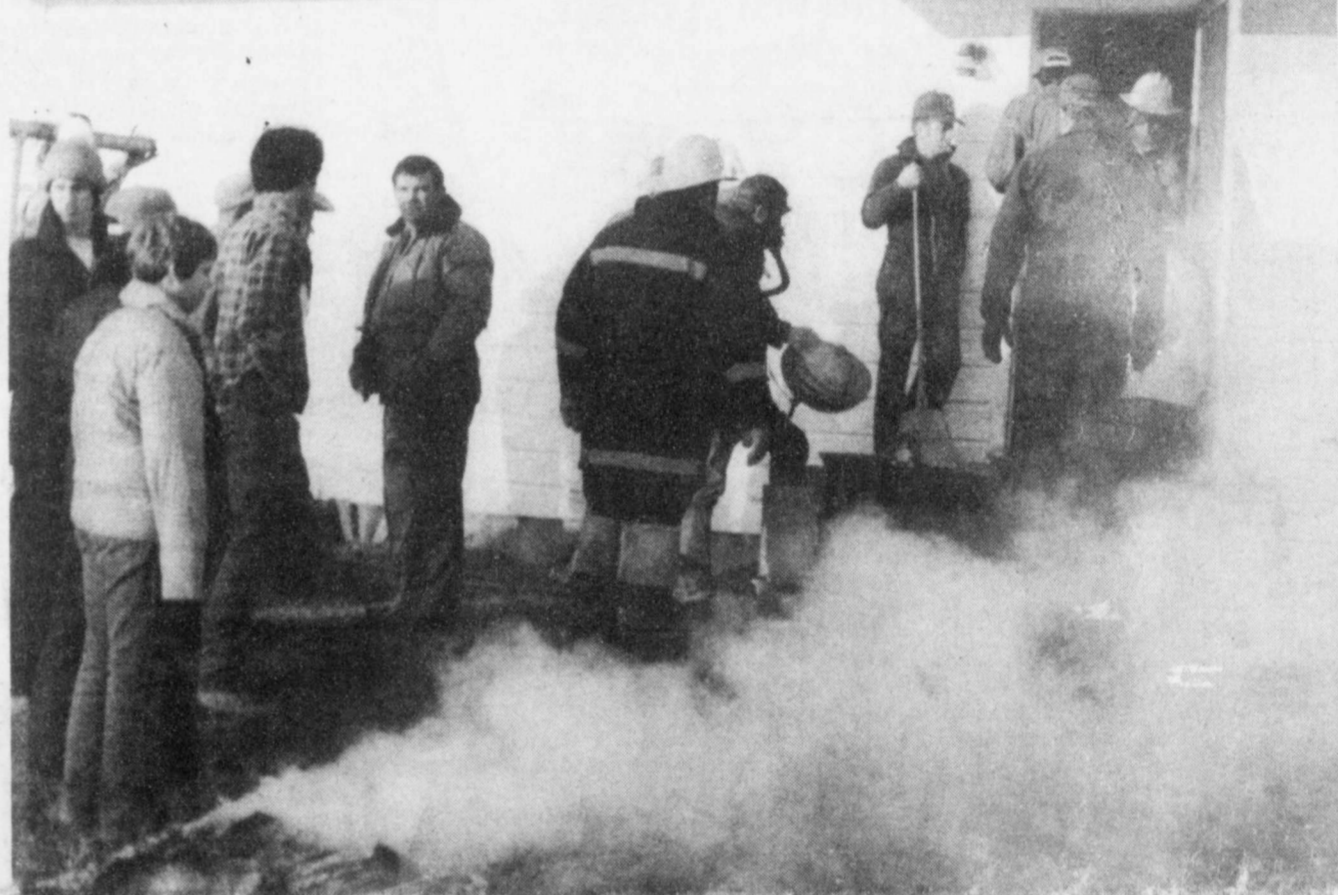
DAMAGE -the home of Bobby Salters was damaged by fire Saturday, when the bedroom of the house caught on fire, apparently from an iron. The bedroom sustained heavy damage. Blossom, Deport and Pattonville fire departments answered the call. (Staff Photo)
