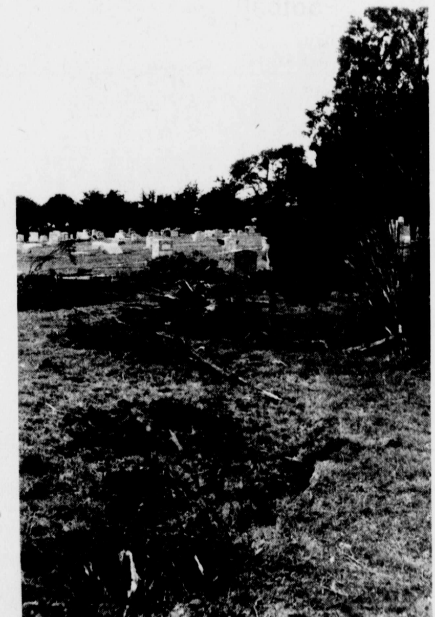
DESTROYED -This large evergreen tree at Highland Cemetery was completely uprooted and torn apart as a vehicle left the cemetery roadway and hit it head on. Another shrub was heavily damaged and the ve-
