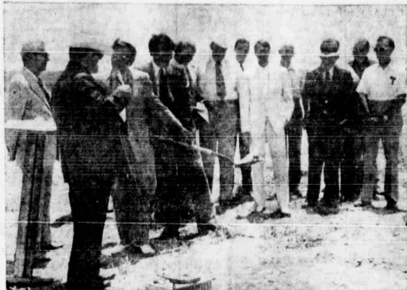
A LOT OF HAPPY FACES show the reactions to groundbreaking activities Monday afternoon at the industrial site of the new Herman Marcus plant. Pictured are, left to right: Mayor Belton Duncan, Haskell Industrial Foundation president Royce Adkins, Herman Marcus, Kenneth Marcus, Barry Henry of Hank Dickerson, R. W. Herzen, Royce Williams, Larry Camp of Camp Construction, J. B. Gipson, Herman Rieherd, of Rieherd & Huckaby, publisher Bill Comedy and Bob Beauchamp. (Staff Photo)
