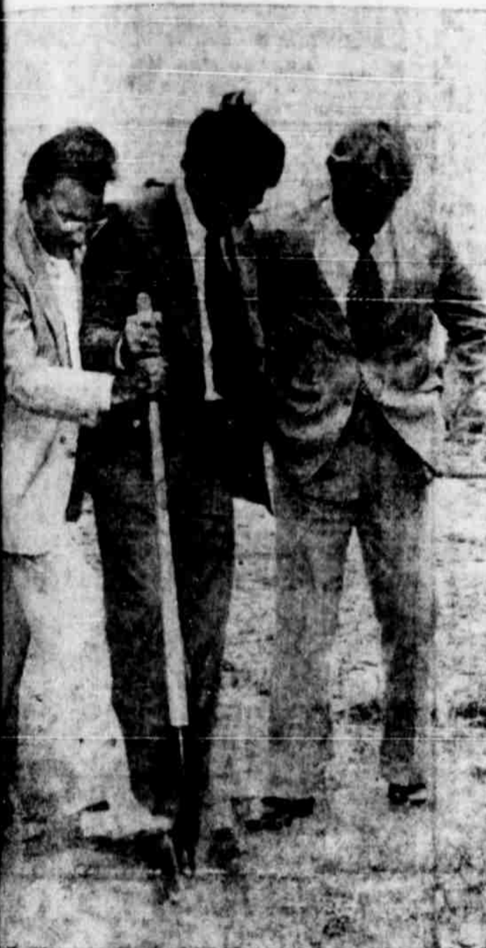
GROUND BREAKING on the new Herman Marcus, Inc., garment plant in Haskell took place Monday, with left to right: Herman Marcus and Richard Marcus of HM, Inc., and Barry Henry of Dickerson Industries of Dallas, turning the first spadeful for the 11,000 sq. ft. building to house the plant. (Staff Photo)
