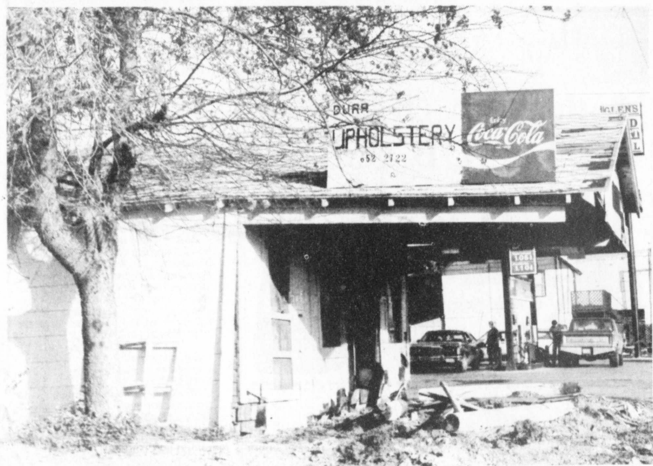
OLD STORE-Pattonville's old store building is coming down now. It is only one of dozens of
