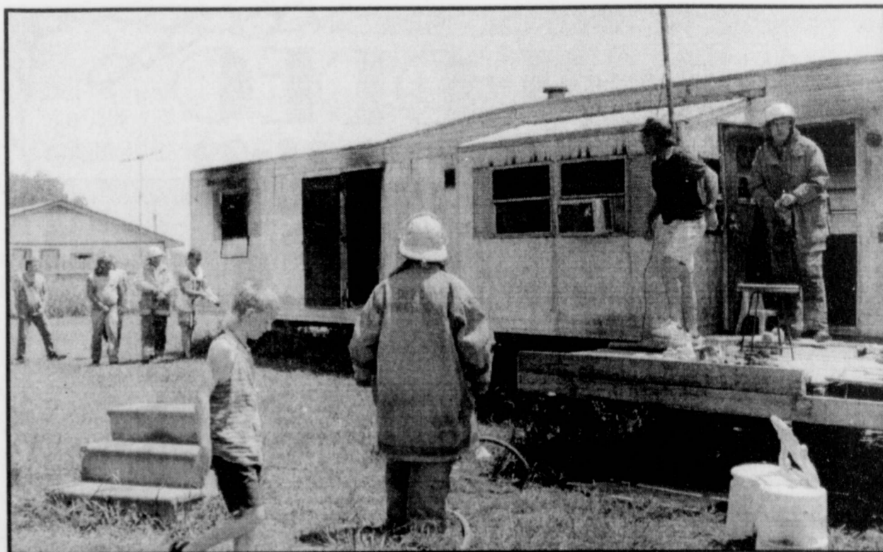
HEATED FIRE -Pattonville and Deport Volunteer Firemen responded to this mobile home fire near Pattonville Monday afternoon. Firemen suffered from the high temperatures of the fire and the weather. The Structure received heavy damage. It is the residence of the Randy Browns, and no one was home at the time of the blaze. Cause of the blaze is unknown at this time. (Staff Photo by Nanalee Nichols)
