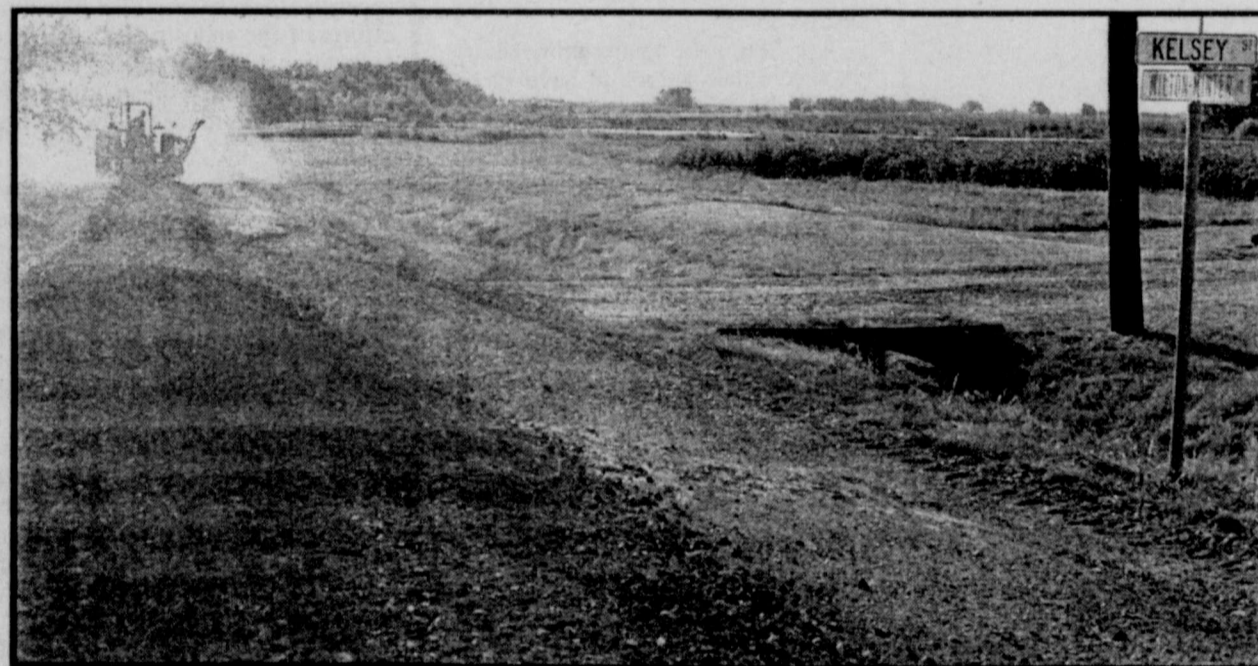
RESURFACED- PCT.. One workers have been helping resurface the Milton-Minter road this week. The new surface will be gravel mixed with oil dirt. (Staff Photo By Thomas Nichols)
