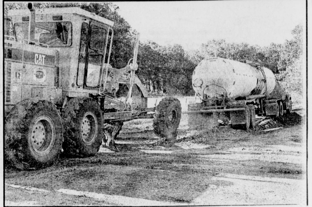
NEW SURFACE-Lamar County Pct. 1 Commissioner Mike Blackburn has had the road crews busy converting several gravel roads to oil surface in the Deport area. The Commissioner's goal is to oil all 300 miles of county roads in Pct. 1 as time and money allows. (Staff Photo by Thomas Nichols)
