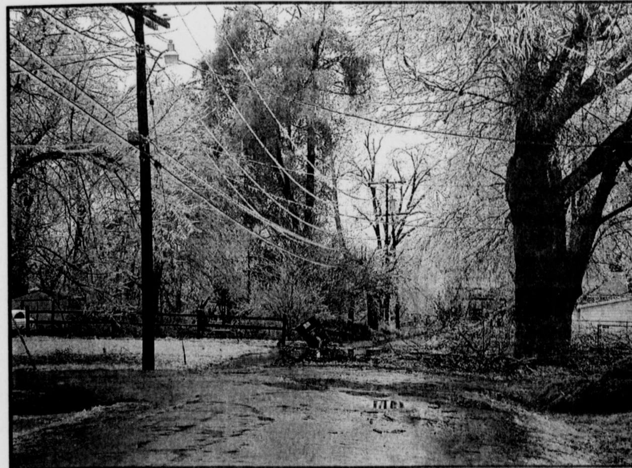
ICY POWER LINES-these power lines, lowered by ice and beset by fallen limbs, are an example of some of the problems the power companies have had to face since the worst ice storm in memory devastated the area last week. (Staff Photo by Thomas Nichols)
