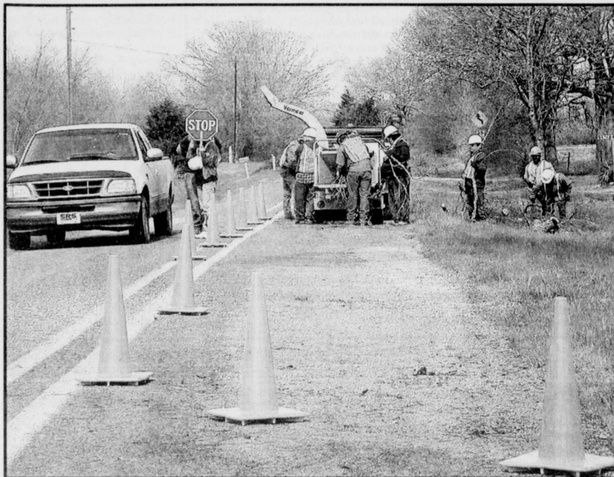
CUTTING AND CHIPPING -Road crews in all areas have been busy on county roads cutting up and hanging limbs and chipping them up. It will take months to finish up with the damage the ice storm that began Christmas Day caused. (Staff Photo by Nanalee Nichols)
