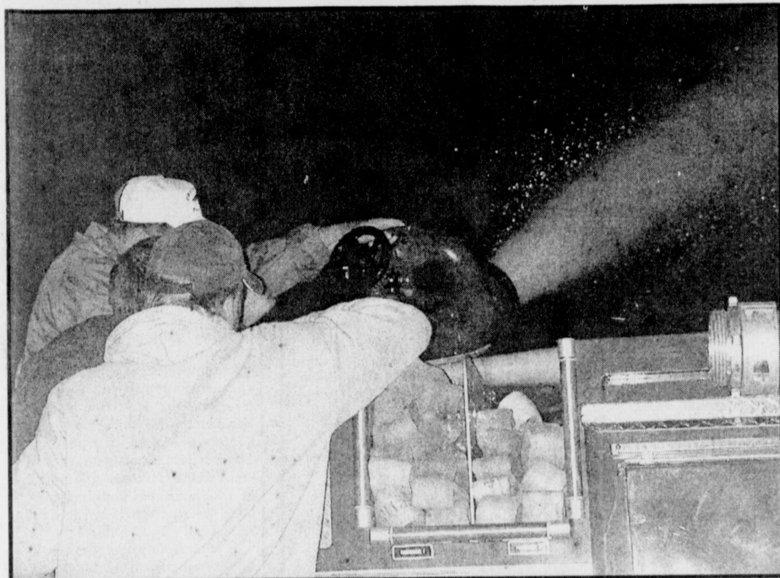
DECK GUN—a powerful new weapon against fire has been purchased by the Deport Volunteer Fire Department. A deck gun was mounted on a fire truck, and should help making fighting structure fire more efficient and safer. The firemen practised with the new apparatus at their last training meeting. (Staff Photo by Nanalee Nichols)
