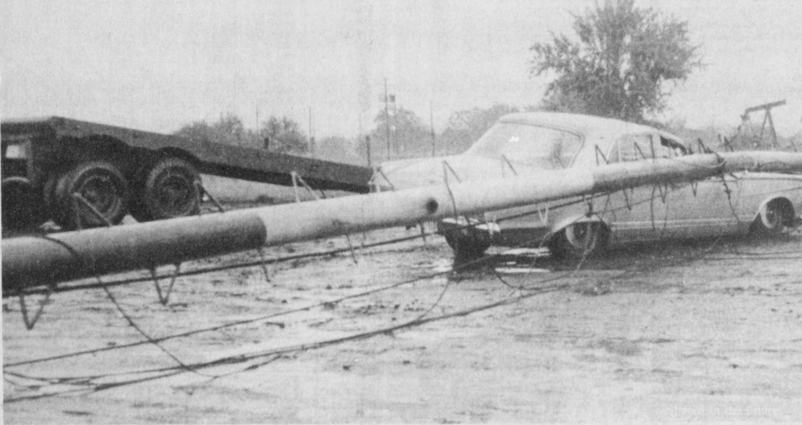
ANTENNA--A 149 foot two-way radio antenna crumbles as storm winds
