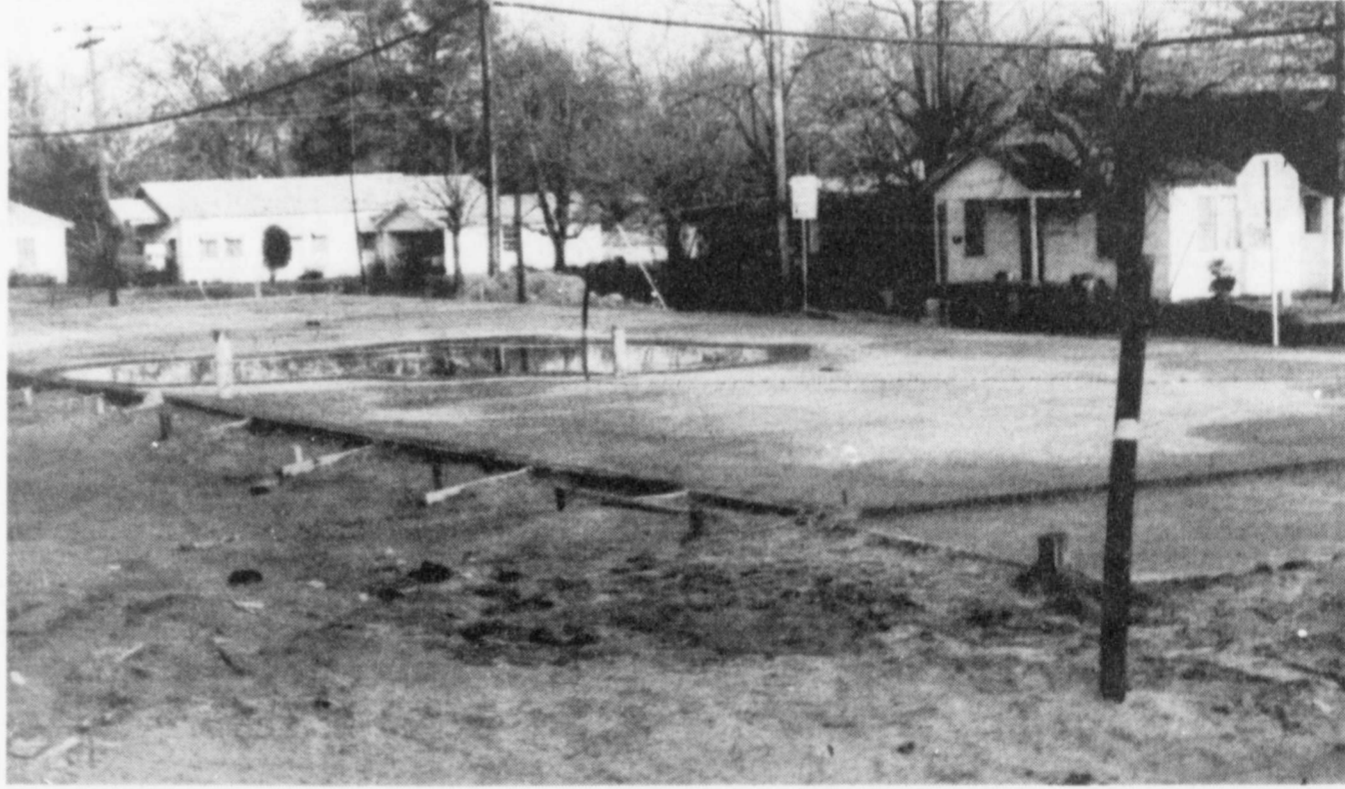
FOUNDATION POURED—The foun- dation for the new
