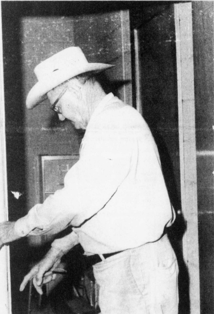
J.N. LEE inspects the door leading into Bogata City Hall that was kicked in some time over the
