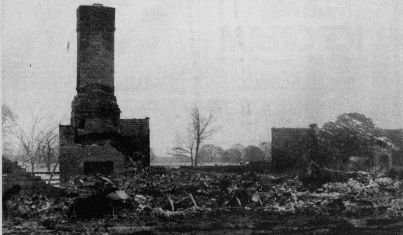
COMPLETELY DESTROYED-this brick home, belonging to Dean and Barbara Ward of
