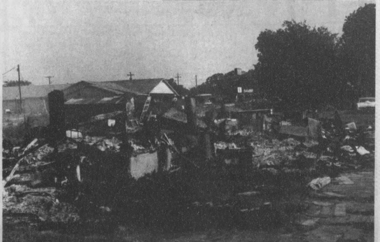
DESTROYED—The Bobby Martin home in Bogata at 2nd St. S.W. was destroyed by fire
