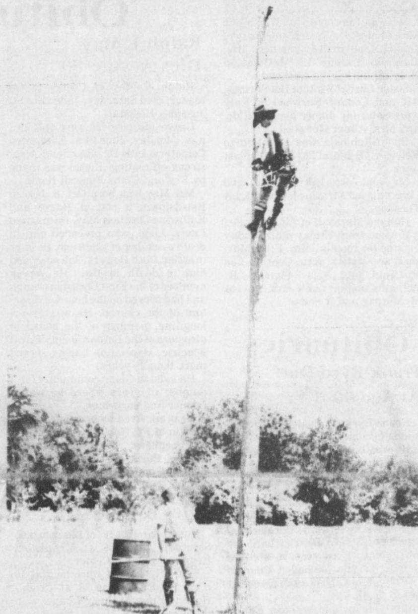
A NEW TV Cable being put up in Talco by Northeast Texas Cable Construction Co. Owners
