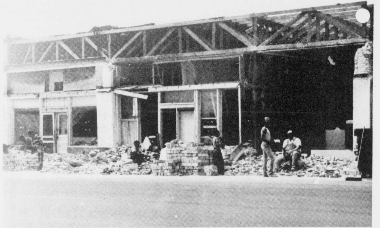
TEARING IT DOWN-The northwest end of Bogata is being demolished to make room for the new Bogata Post Office. The old brick buildings are disappearing fast! (Staff Photo by Diana Eudy)
