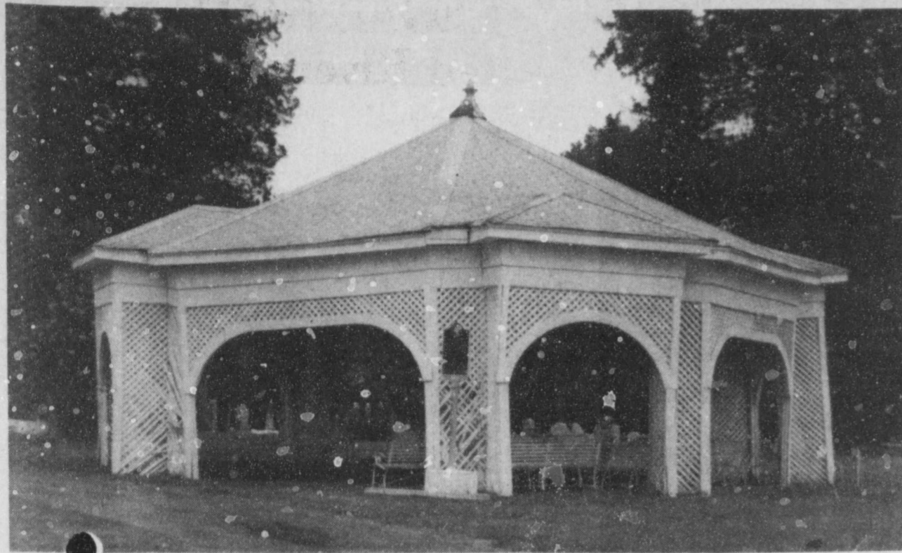
THE HISTORIC pavilion at the Bogata Cemetery is badly out of level and in desperate need of
