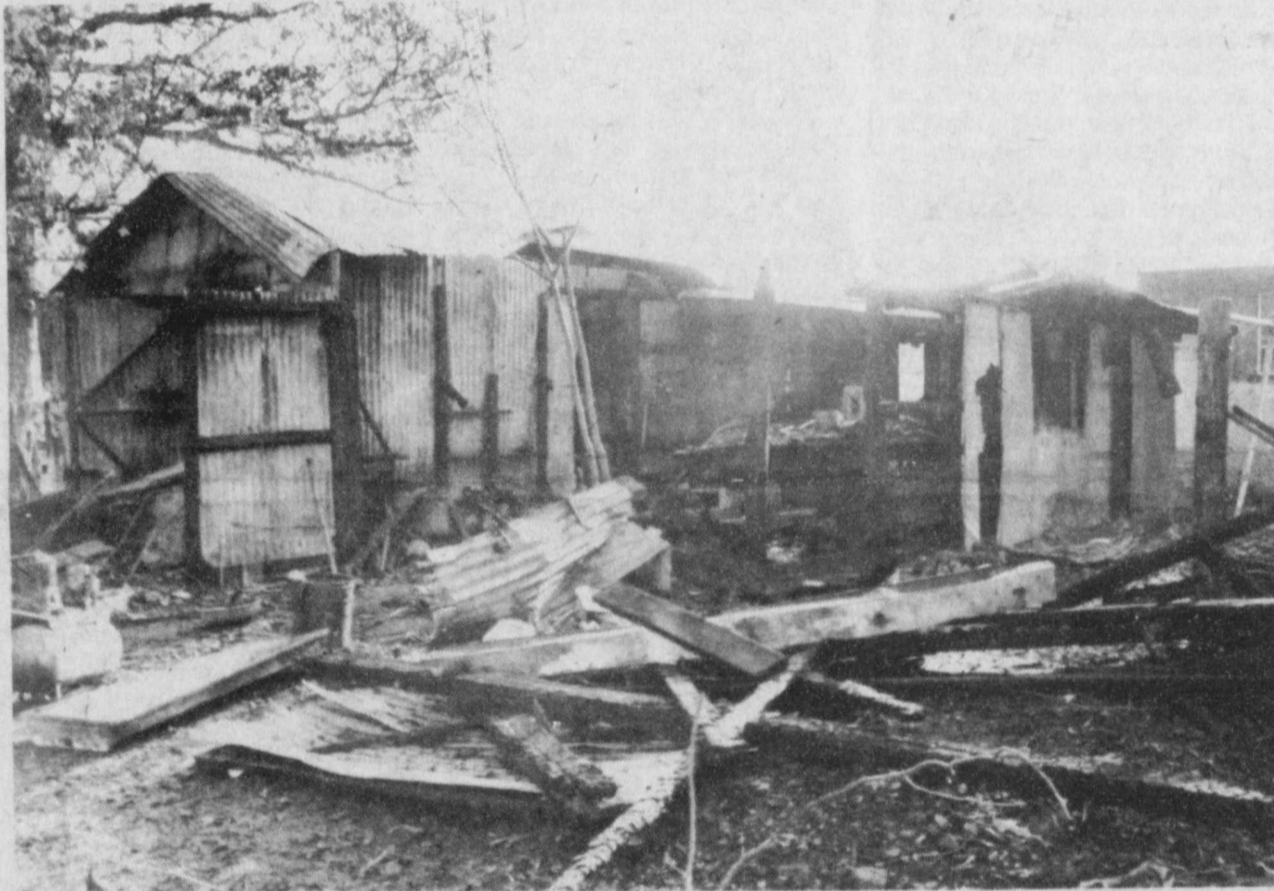
THE CHARRED remains of Russell Woodall's small engine repair shop are the result of a fire which totally destroyed the structure Thursday night, January 26.
