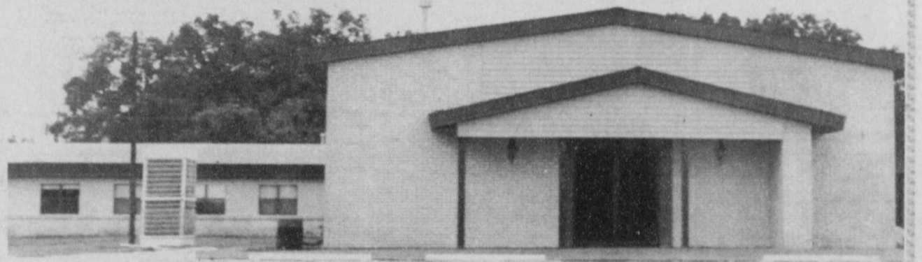
CALVARY BAPTIST Church in Talco recently received a face-lift and this week the finishing touches were added to the church when the steeple was installed. (Staff Photo by Nancy Brown)
