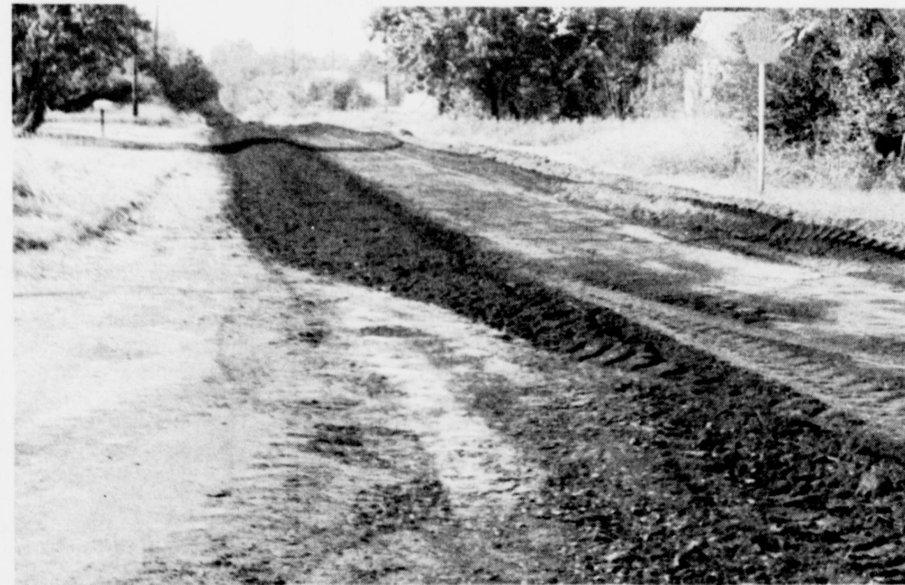
NW 5 and NW 9 County Roads are being reworked this week in
