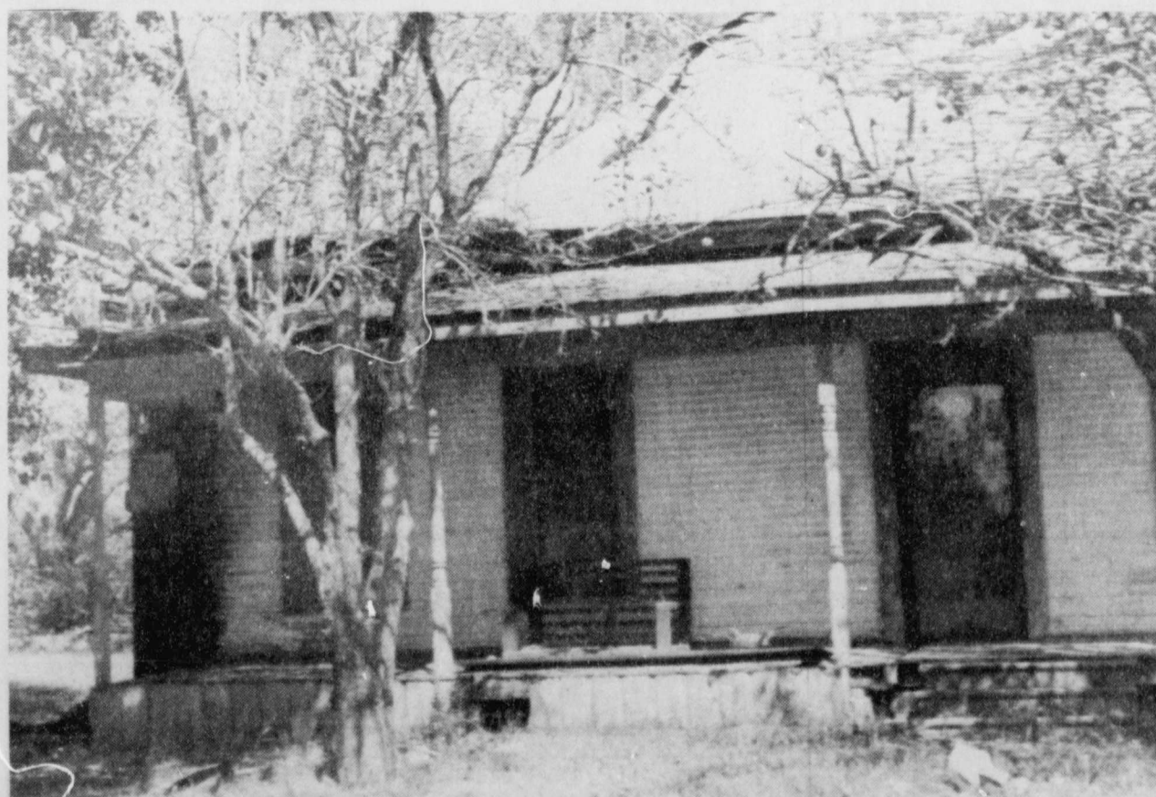
SEVERE DAMAGE--The home of Kenneth and Darlene South-erland was severely damaged
