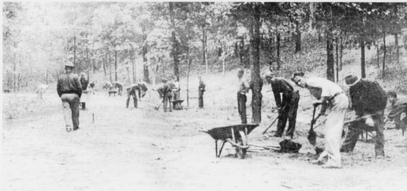
OLD PHOTO-this photograph of the CCC (Civilian Conservation Corps) show road work being done. The CCC was formed during the depression and provided work plus conservation efforts. This photo shows a roadbed being leveled with shovels and hoes.
