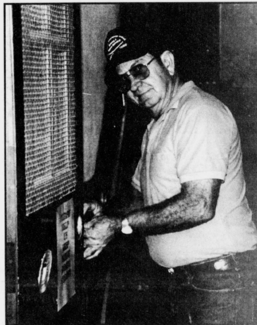
BREAK IN-Talco School was broken into sometime during the night Wednesday. A glass was broken in the office and the door to the cafeteria was damaged. Pictured is Blanton Gage of the Talco-Bogata CISD Maintenance as he repairs some of the damage. Nothing could be missed in the school. Mr. Gage did not know he would be called again on Sunday when the school was again broken into. Sometime between 1-2:00 p.m. Sunday afternoon person or persons broke into the school this time doing major damage. Over eight windows were broken, the candy machine was destroyed for the change but little candy was taken, the office, gym, class rooms and lockers were broken into also. Change from the candy machine, small amounts of money was taken from the teachers desk, Halloween stickers, a set of keys and several other small items were missed. The Mt. Pleasant Police took finger prints from the coke and candy machines and they did have suspects in the case. At press time no charges had been filed. (Staff Photo Nancy Brown)
