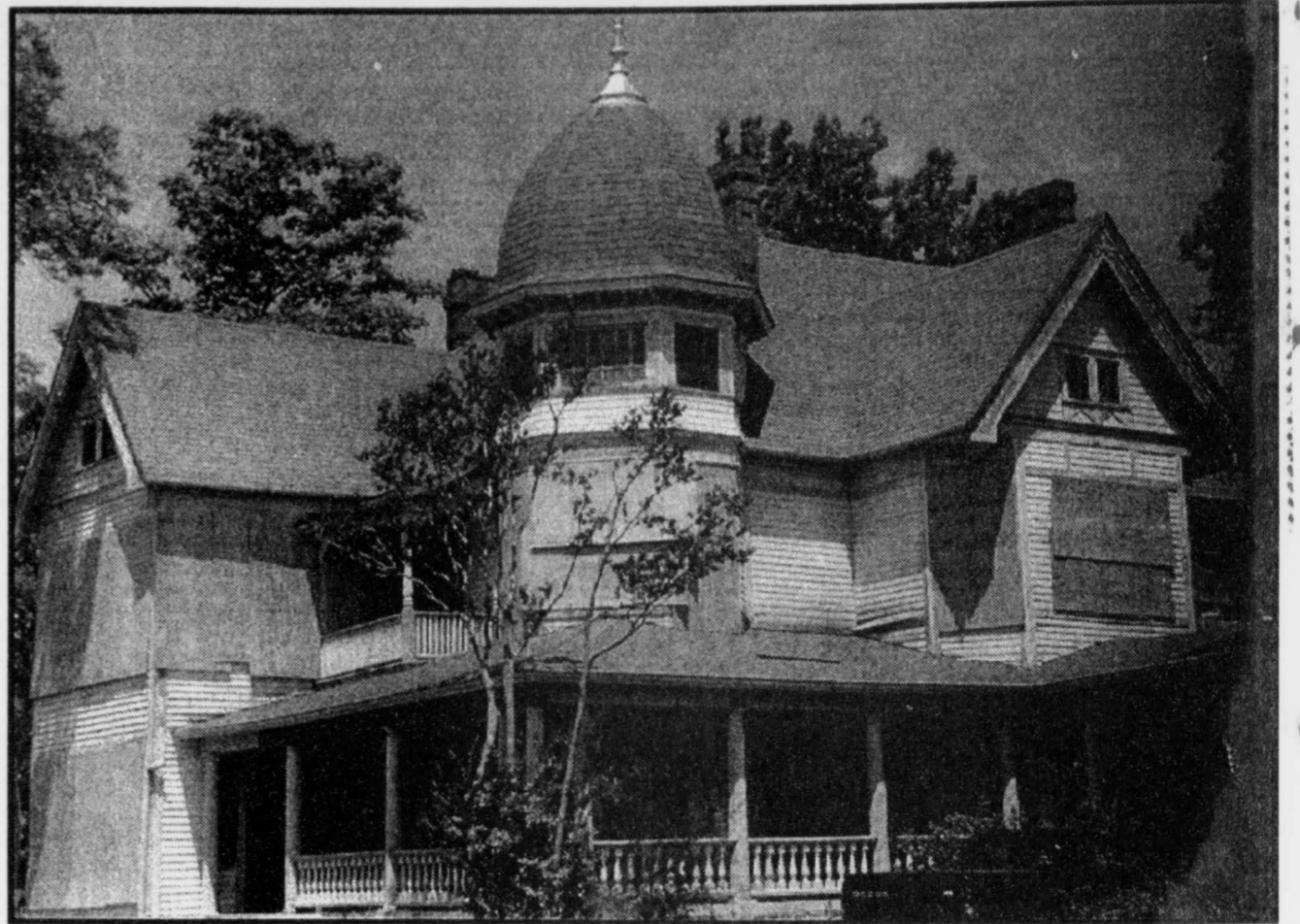
WORK IN PROGRESS -The Red River County Historical Society is in the process of restoring the Lennex home in Clarksville. According to the Historical Society President Jack Herrington the project is expected to be completed by the end of the year. President Herrington purposes the house be used for special occasions such as service clubs, weddings and etc.
