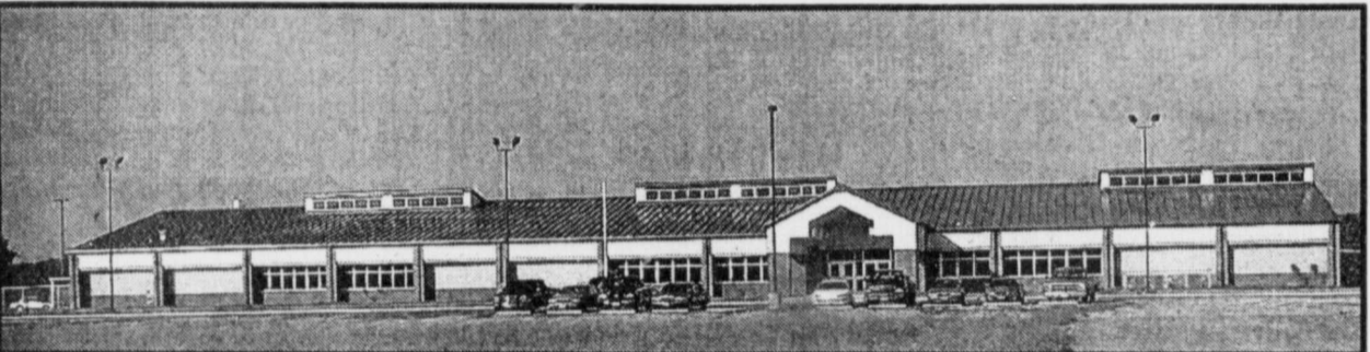
ALMOST READY-Teachers and staff of the Rivercrest School District were busy this week moving into the new elementary school located on Hwy. 271 near Rivercrest High School. The school will hold an official open house soon. (Staff Photo Nancy Brown)
