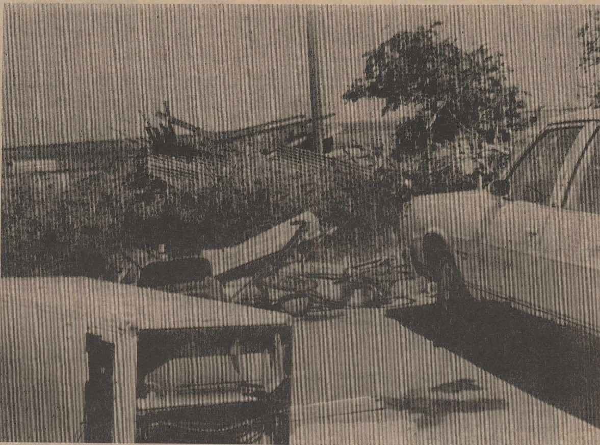
The shop and garage building was completely destroyed by the storm that came through the area Monday, on the Guinn Fitzgerald farm
