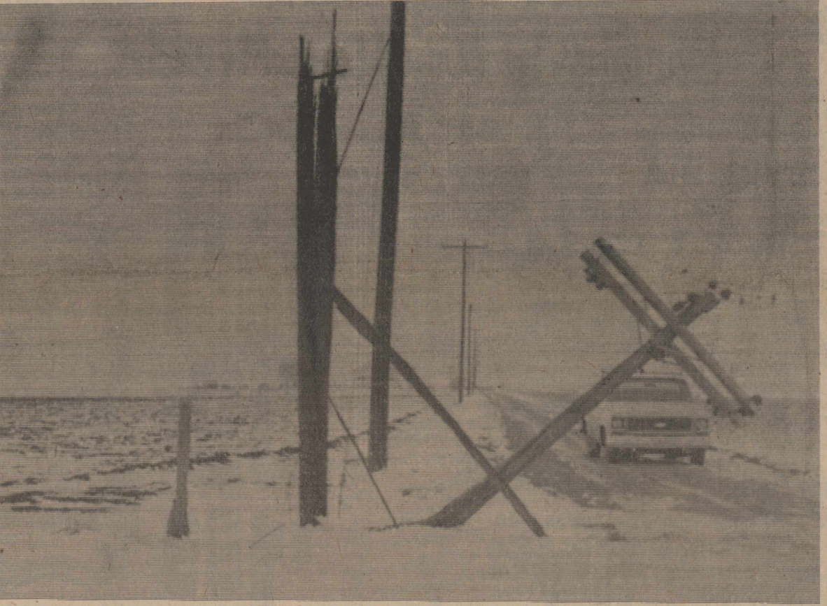
Like dominoes they went down! Ice on utility wires the size of a man's arm brought utility poles down at the Glen Lindsey farm northeast of Silverton. Most resi-
