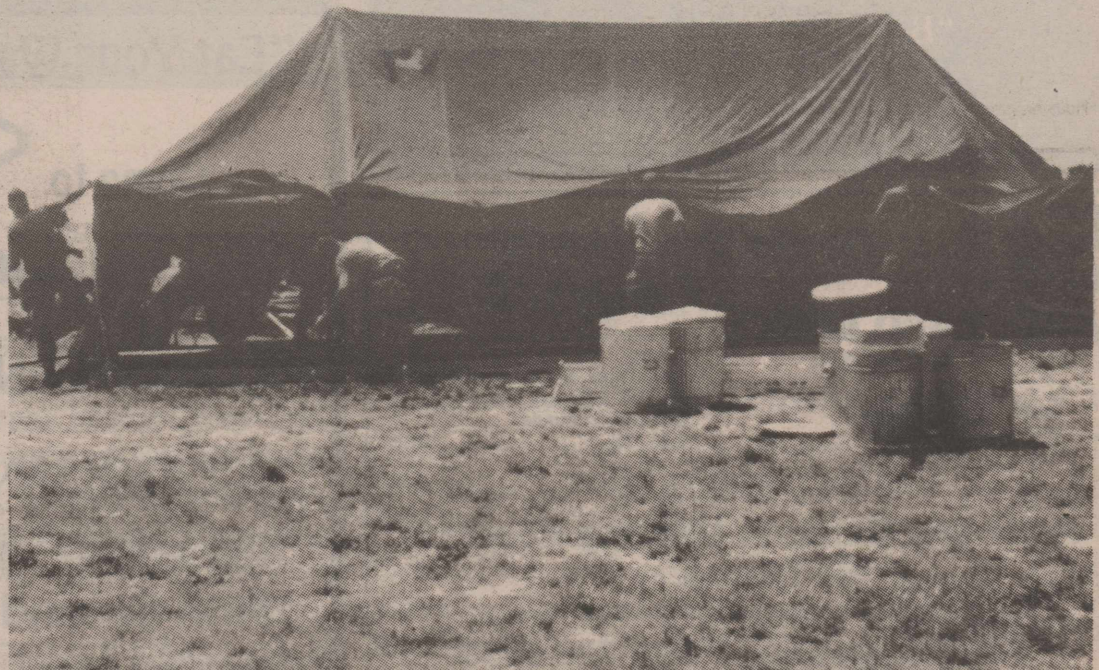
One of the 17 tents erected by civil engineering.
