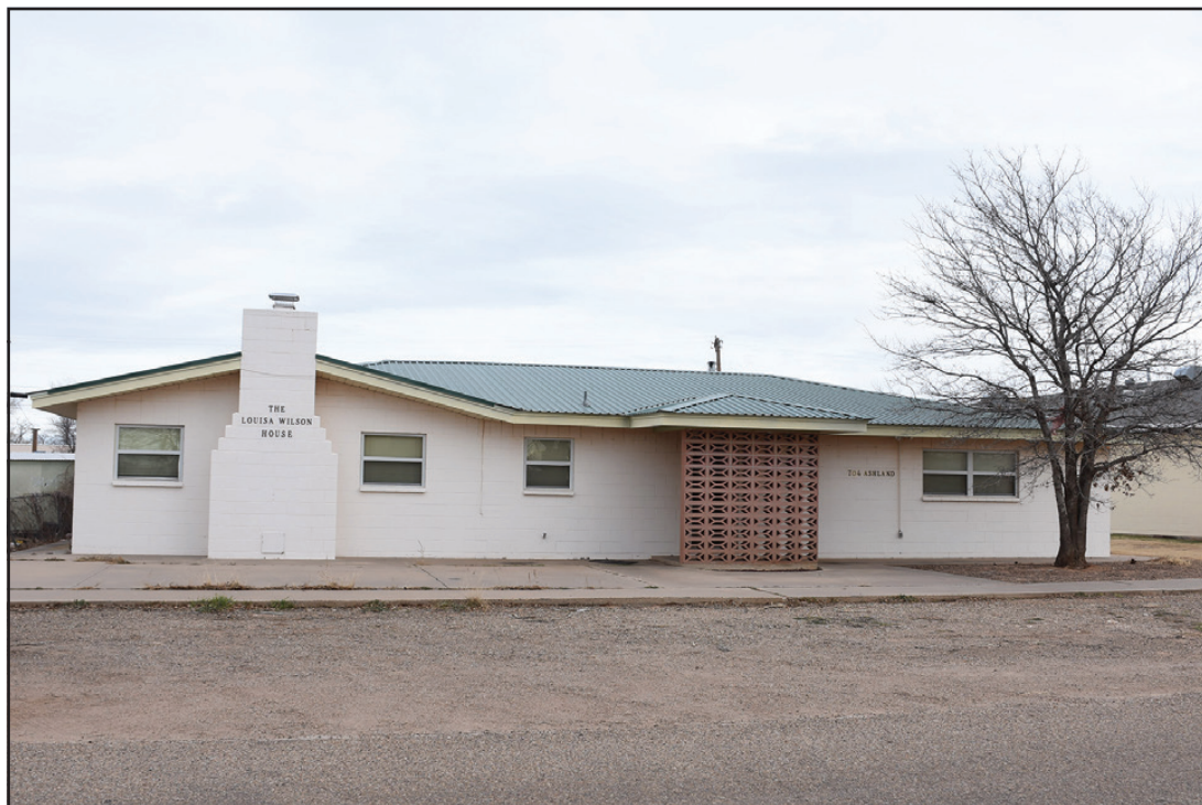
Old Girl Scout Building (The Louisa Wilson House) at 704 Ashland
