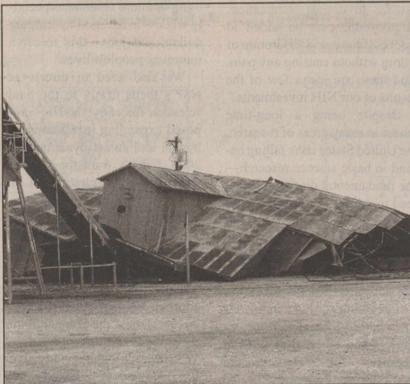
South side of warehouse in Rochester
