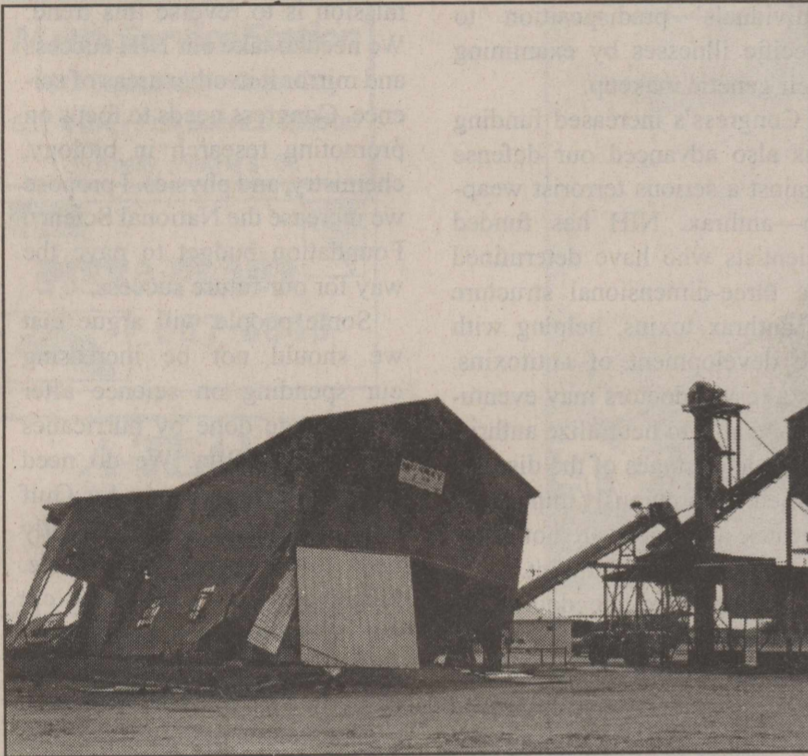
West side of Warehouse in Rochester
