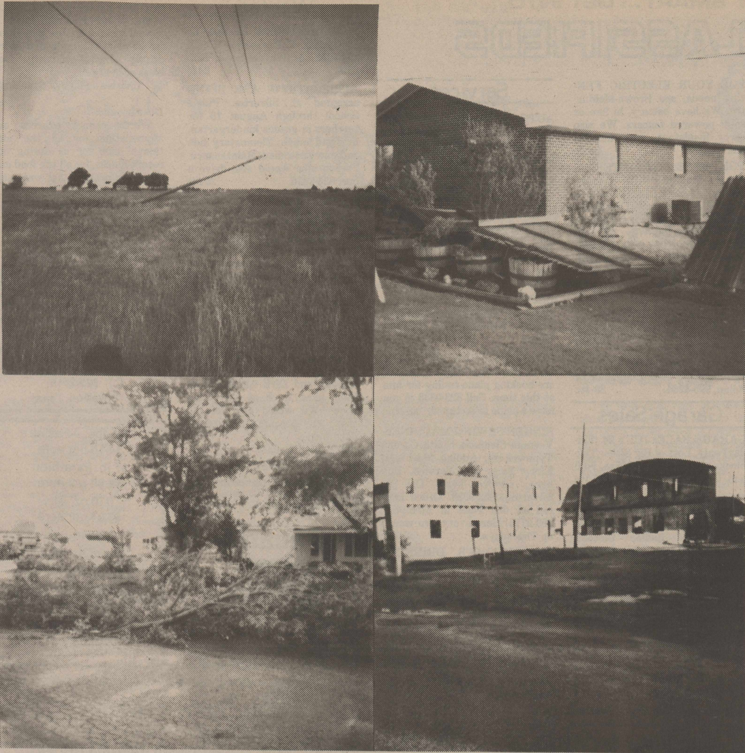
Silverton residents have been assessing the damage done during a severe hail, wind and rain storm which swept across Silverton on Tuesday night of last week. Pictured is a power pole that was toppled east of the Cam Forbes home, the fence between the George Seaney's and Charles Sarchet's, and tree limbs at the Edwin May home. The east wall of the old Burson building was blown in, roofs and vehicles were damaged and windows were broken.
