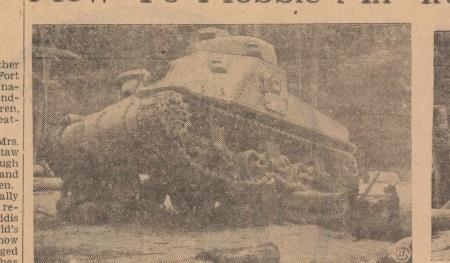
A tank goes over a "ramp" obstruction, designed to cut down speed before it hits the "stopper" crib of logs. Note how ramp forces tank's forepart up, exposing vulnerable belly to anti-tank fire.
