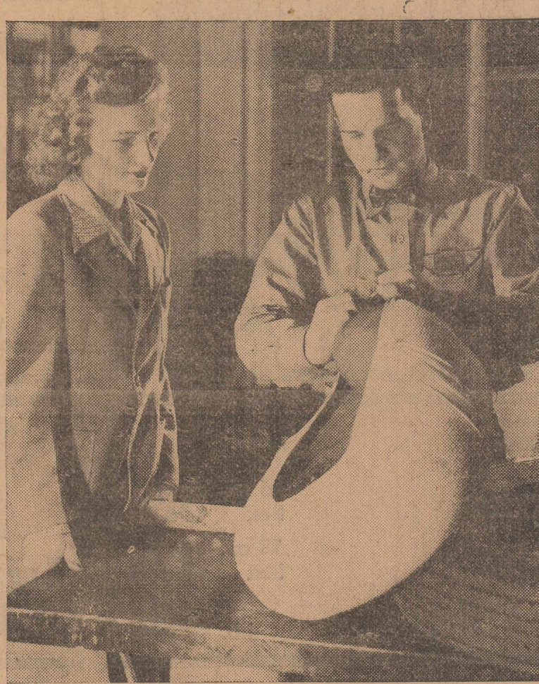
This is how Firestone's new cotton "girdle" for inner tubes is applied to a tube which is going back into service in a tire which would ordinarily be unfit for use because of body cuts and breaks that would chafe through the tube in a few miles of driving. Miss Dorothy St. Lawrence of Providence, Rhode Island, a trainee for a Firestone Store Managership, sees the step-by-step procedure that will return to service a tire hitherto condemned to the scrap pile.
