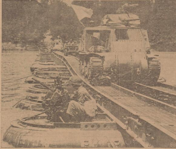
(U. S. Army Signal Corps Photo from NEA) Passing over a machine gun-guarded ponton bridge, a big U. S. tank makes the structure sag a bit, but goes safely across. Behind it come a jeep and another tank on maneuvers demonstrating use of pontons for crossing rivers where bridges have been destroyed.
