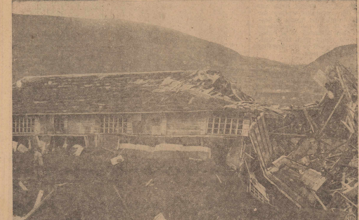
Indication of why the Japs left Kiska is seen in this demolished airplane hangar that was hit during the U. S. air and sea bombardment of the island when it was in enemy hands. American and Canadian forces occupying Kiska found nearly all enemy buildings in this general shape.
