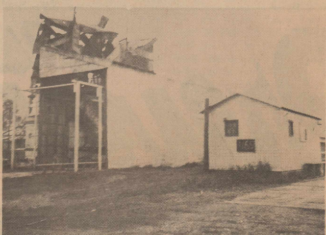
THE MORNING AFTER: The fire was said to have started in the top of the grain storage elevator while a truck was loading at approximately 10:45 Tuesday night.
