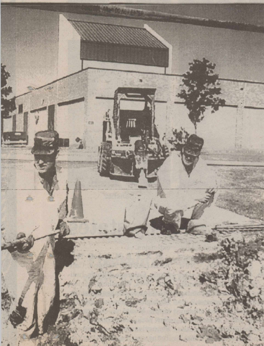
tz dig a ditch. The two members of the operations flight are replacing a water line.
