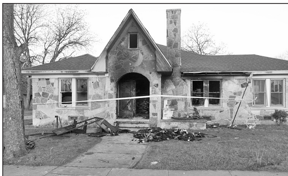
HOUSE FIRE-Mon., April 6 at approximately 9 p.m., members of the Haskell Volunteer Fire Dept. answered the tones to this house fire at 107 N. Ave. C in Haskell. The home of the Seeliger family suffered both fire and smoke damage. The cause is under investigation.
