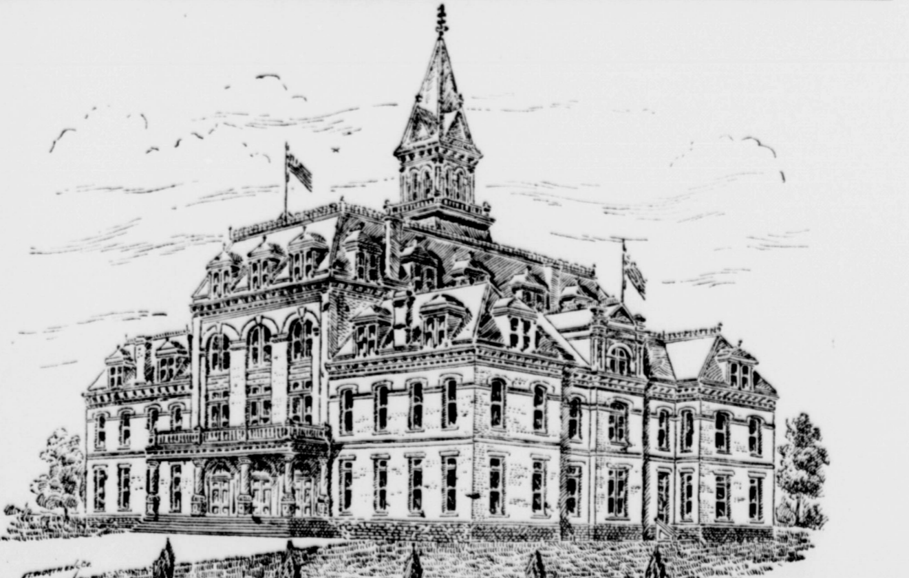
(Plan of building adopted. The right wing is completed, and the rest to be completed as soon as practicable.)
