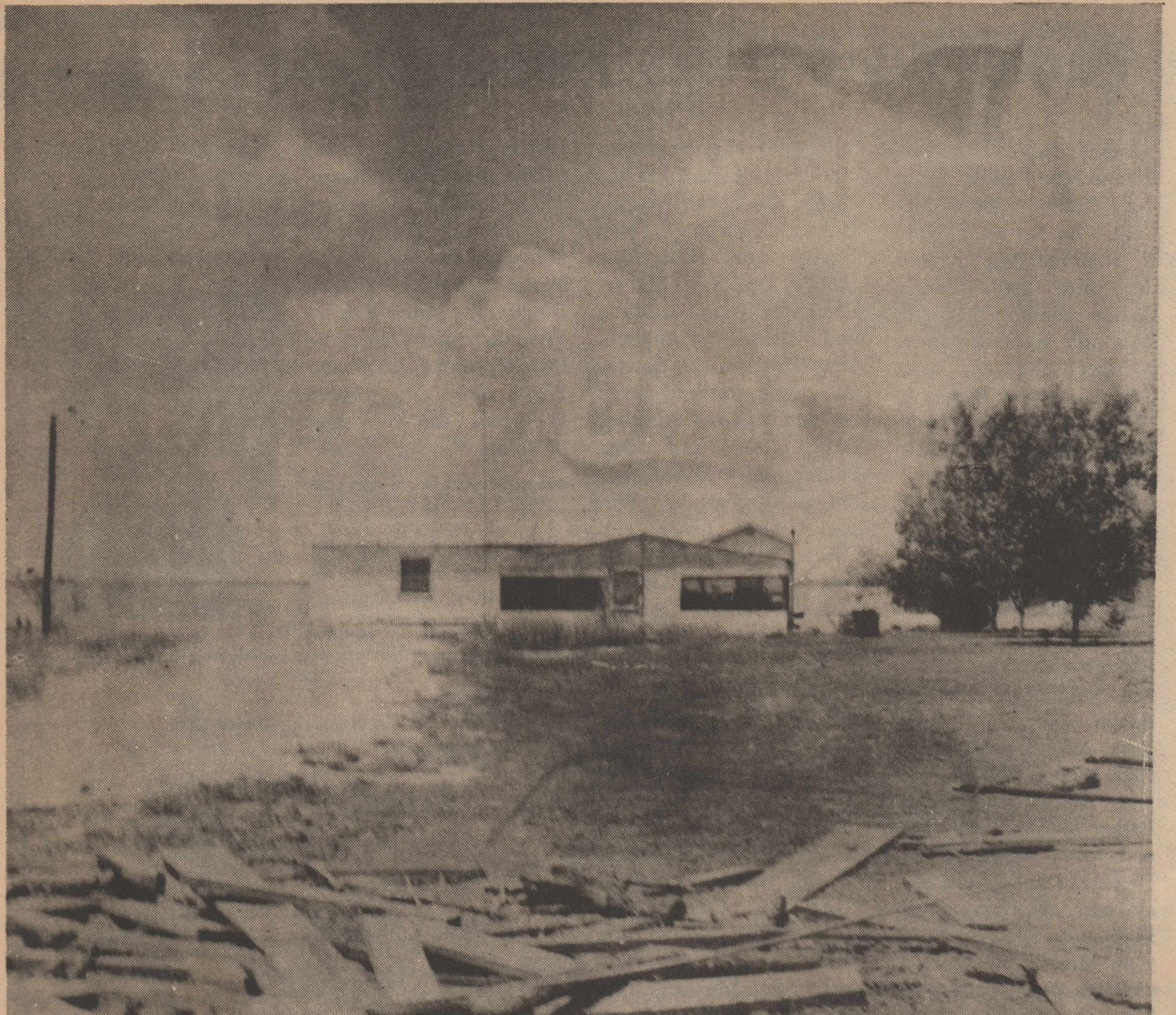
STAMFORD LAKE CABIN: The above picture taken late last Sunday afternoon of the Rotan Firemen's cabin at Lake Stamford, shows only minor water damage compared to other homes around the lake. Rotan Fire man, Archie Neeley, indicated that there was approximately six inches of water in the cabin Saturday. The only damage anticipated will be to the floor. The Rotan Fire Organization has owned the cabin since 1960.
