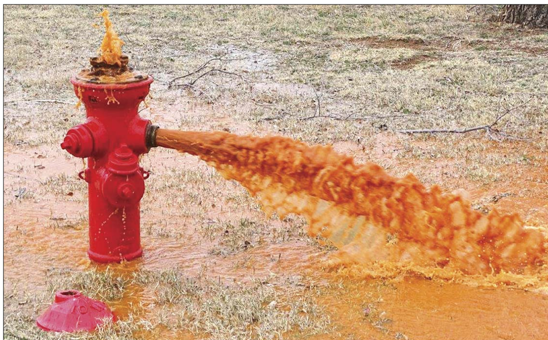
Red water flushes from a fire hydrant near the Saints' Roost Museum as an example of discoloration caused by old cast iron distribution water lines, according to city officials. A Town Hall meeting will be held March 29 to discuss a $3.9 million proposal to address issues such as this. For a map of the proposed project, see page ten.
