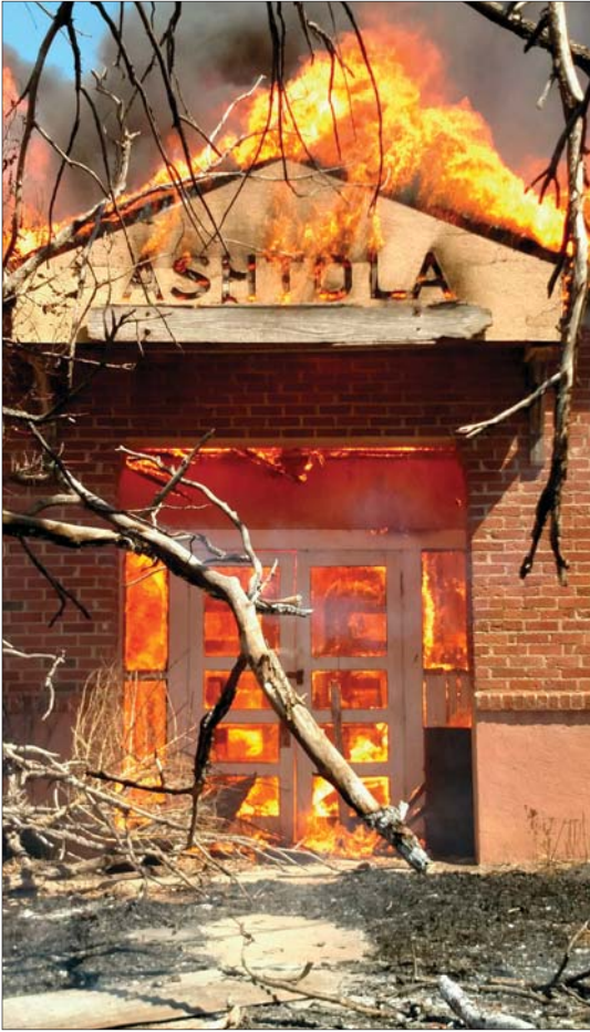
The 1930s-era Ashtola school building was destroyed Tuesday after an accidental grass fire got too close to the building. Clarendon Fire Chief Jeremy Powell is urging all residents to be extremely careful this week as conditions will be right for a disastrous fire to occur. Powell says people should avoid doing anything that might possibly cause a wildfire through this Friday.
