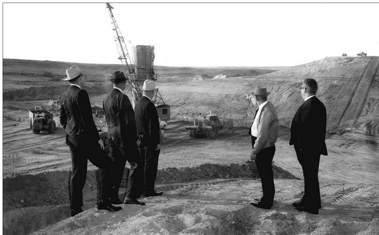
Shown here observing the construction of the Greenbelt Dam are Bill Lowe of Clarendon, Wendall Harrison of Memphis, Merle Kincaid of Crowell, job engineer R.C. Alexander, and Carroll Knorpp of Clarendon.
