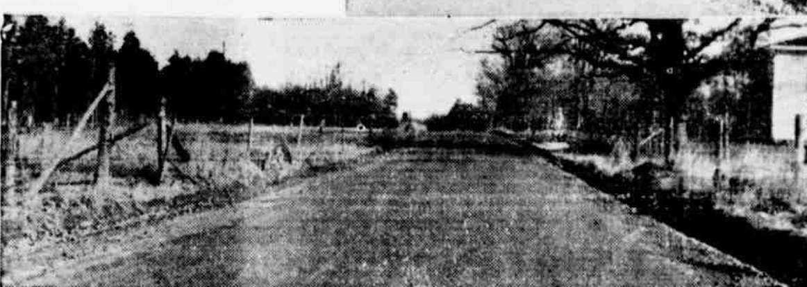
Once not more than a mud road like the one pictured above it, this Virginia thoroughfare resulted from the proper mixtures of local soil materials and calcium chloride to give a "stabilized" turnpike of the type recommended by the U. S. Bureau of Public Roads for low-cost, all-season purpose.
